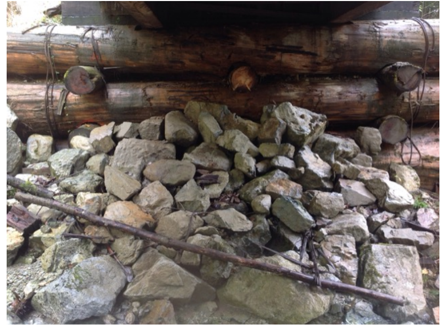
Left Bank Abutment when facing downstream
