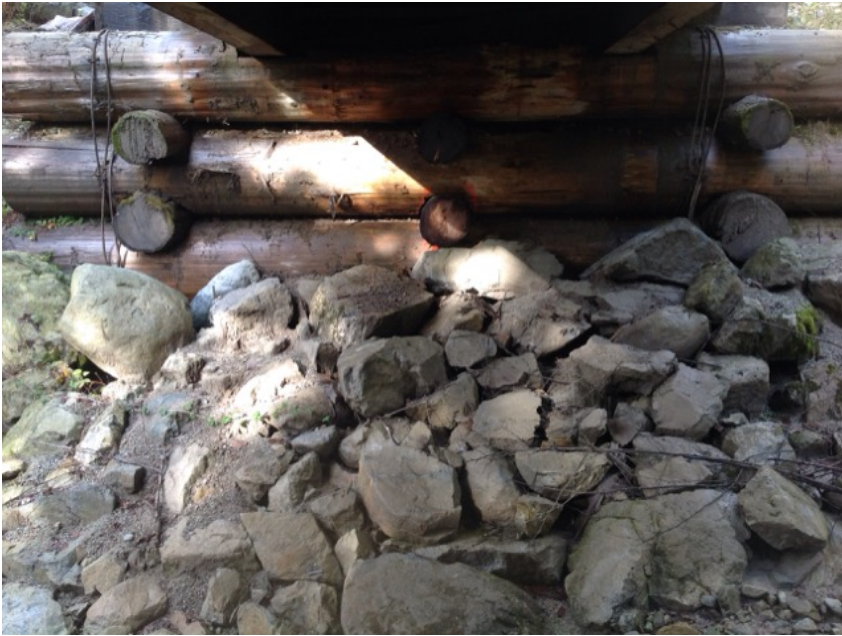
Right Bank Abutment when facing downstream
